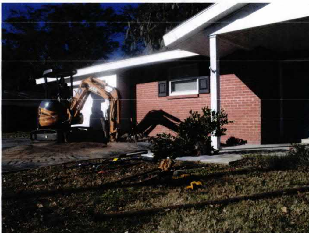
Picture 2: UST 668Camellia excavation in progress.
